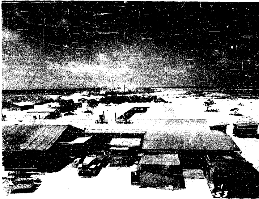
Fig. 3.16 Mess Hall, Tare Island, Preshot
